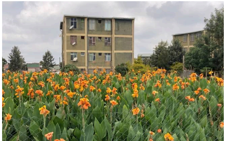
Constructed wetland, Shashemene.
