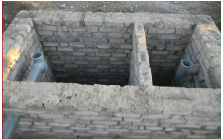
A two-chamber septic tank under construction.
